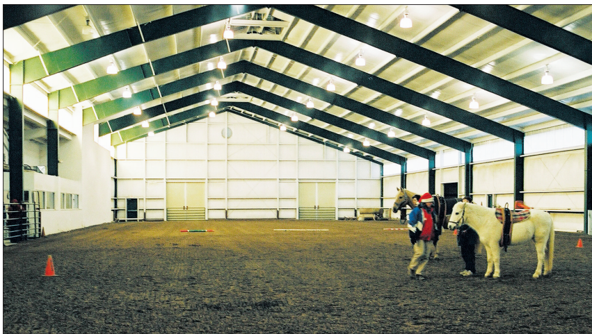
The indoor arena is 225 feet by 85 feet and has a crumb rubber and sand footing. It is unheated but stays about 40 degrees, even when outdoor temperatures plummet.
