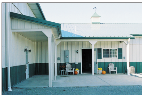
Ann Hamilton hired Morton Buildings to construct the barn, but she served as general contractor on the project.
