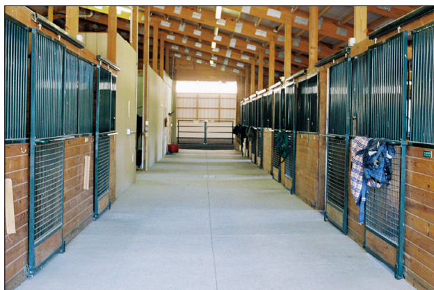
A stall aisle, one of two that run parallel to each other, is made up of 12-by-12-foot stalls. The wash rack area and tack and locker room are in a connecting walkway.
